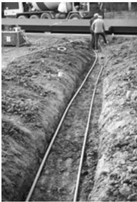
Figure 3-1. Conduit Run in Trench
